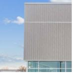
4. FIBER CEMENT BOARD NICHIHA LATURA V-GROOVE OR EQUIVALENT
